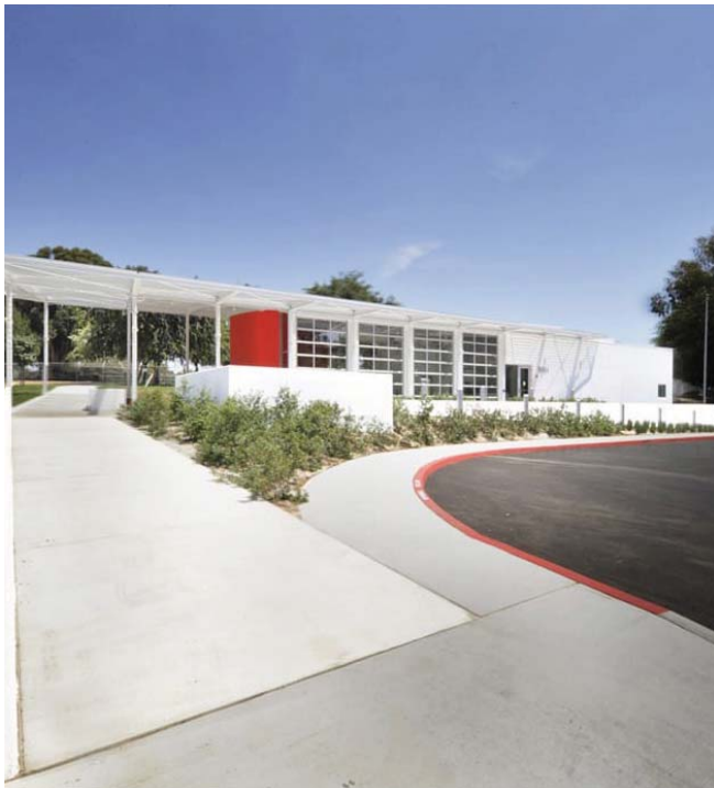
Portero Heights Community & Senior Center Building
