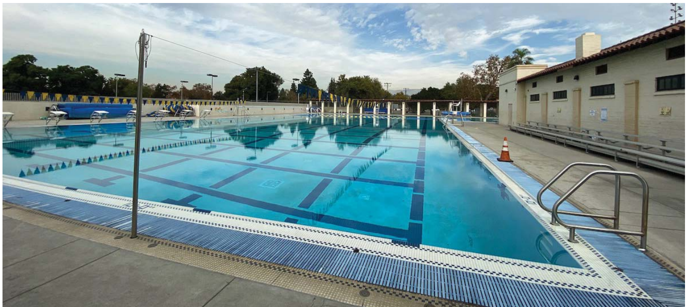
Pool facility at George Hensel Aquatic Center
