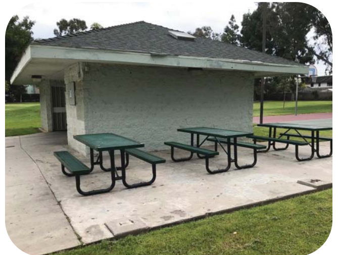
Existing restroom facility at Montebello park
