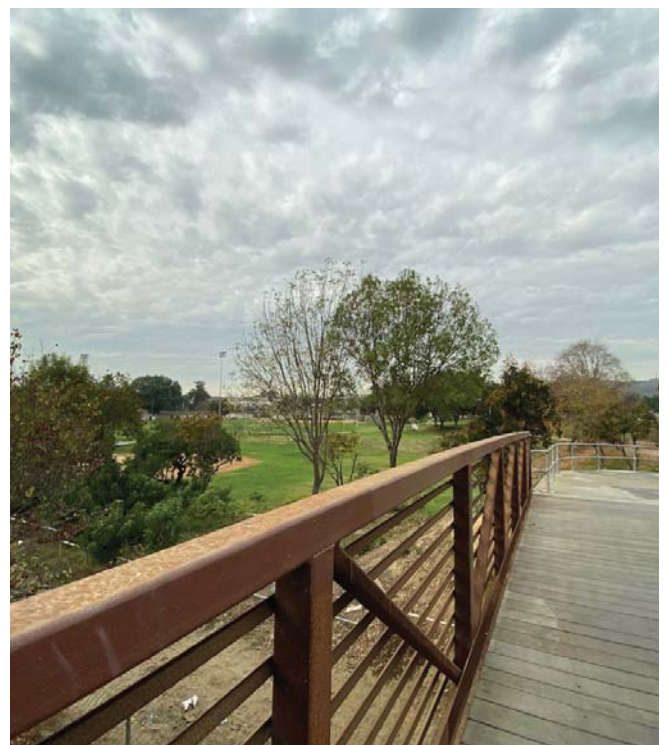
Bridge from Grant Rea Park to Rio Hondo Trail
